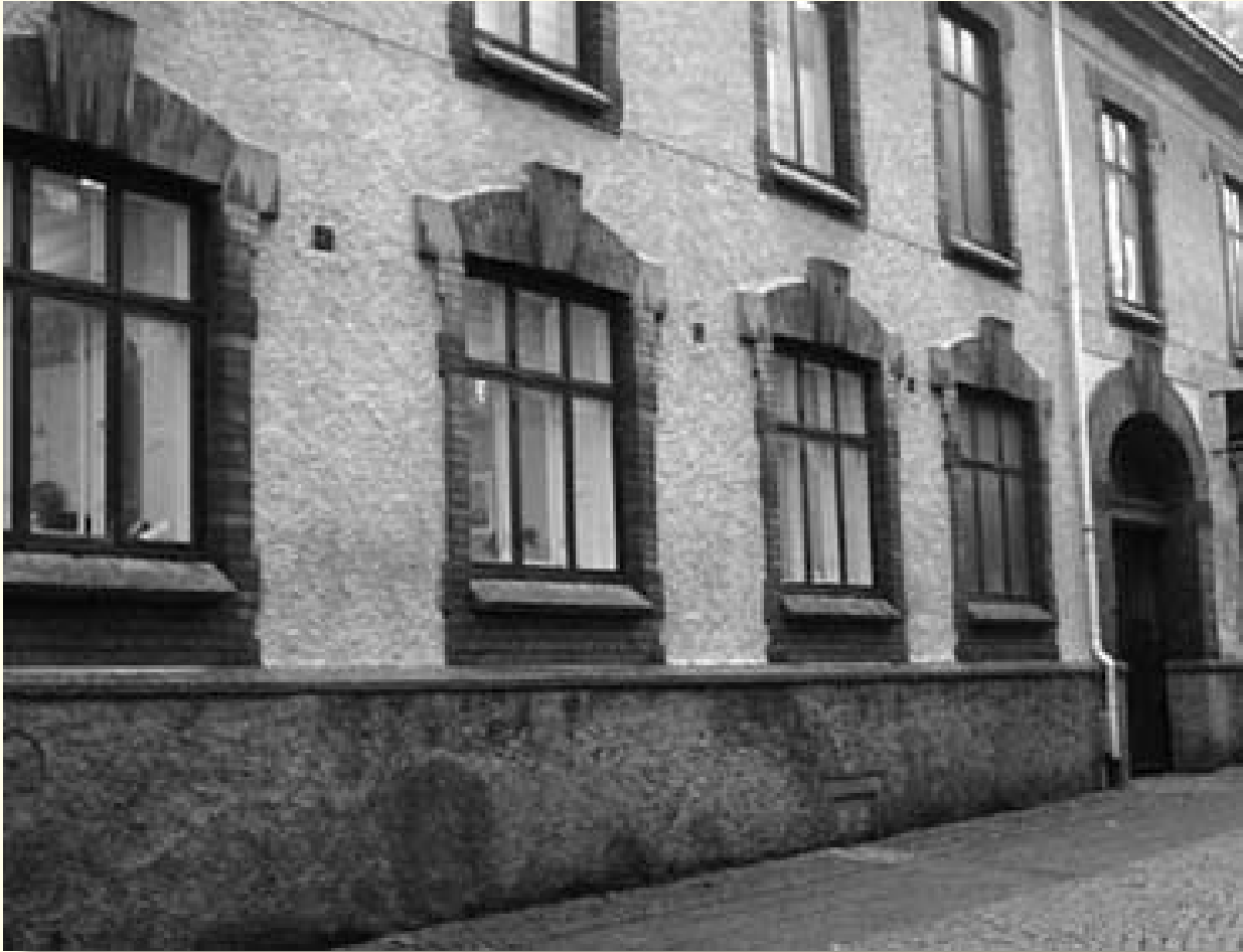
ABOVE: POLICE HOUSE AT LILLA BOMMEN. THE ENTRANCE TO THE BACKYARD IS VISIBLE ON THE FAR RIGHT
